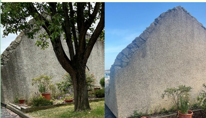
Before & After of the back wall of the Grotto
